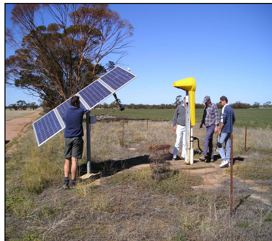
Figure 1. Solar powered groundwater pumping.
